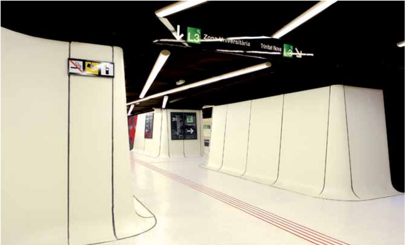
The clean and bright look of the space is achieved through the use of GRC (Glass Reinforced Concrete) panels, which provide the same qualities of reinforced concrete but are five times lighter. The Terrazzo pavement continues throughout the station.
