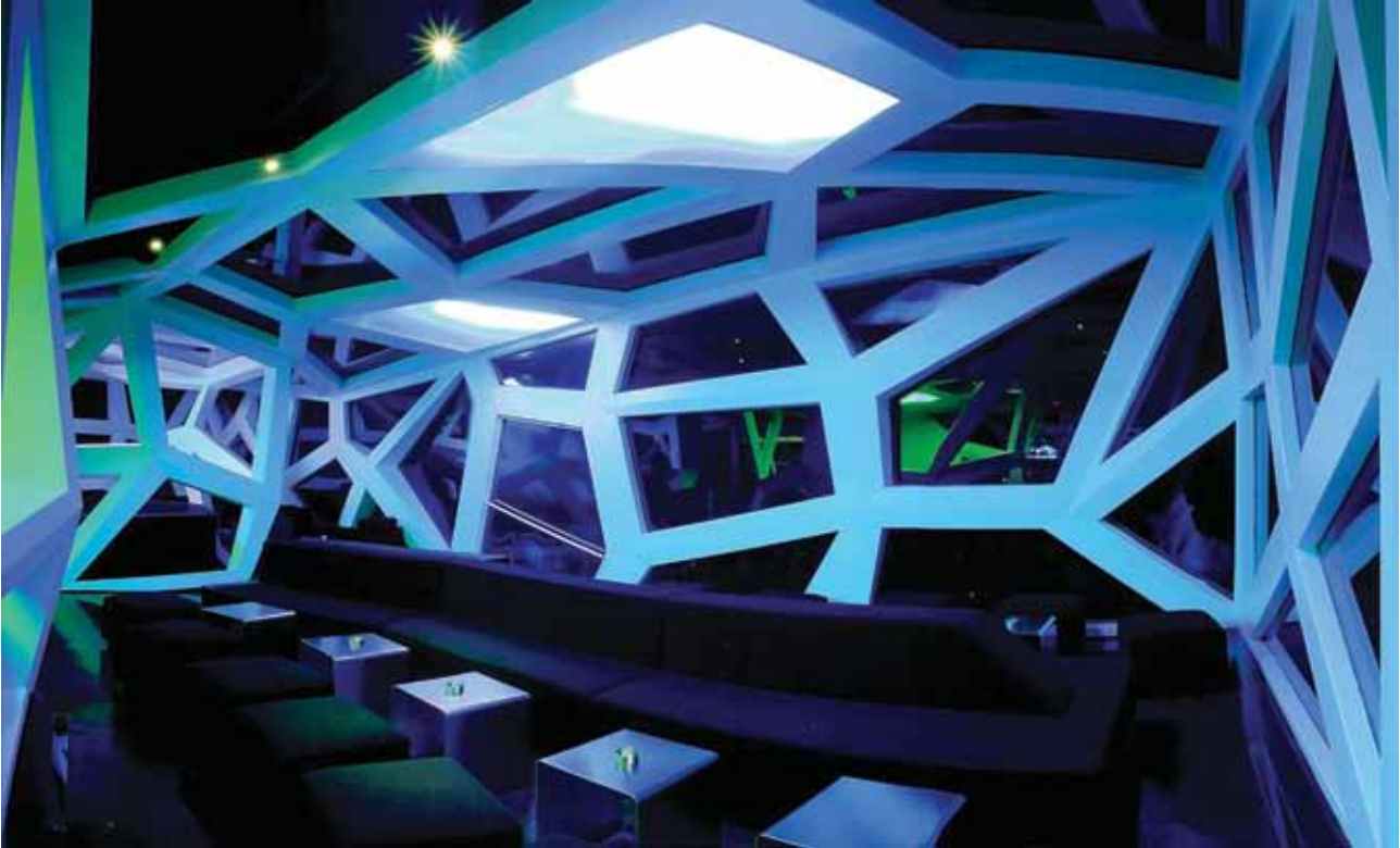
The complex netting of the steel mesh, cut by numerically controlled machines, configures both the exterior glass, composed of different geometries, as well as the interior spaces.
