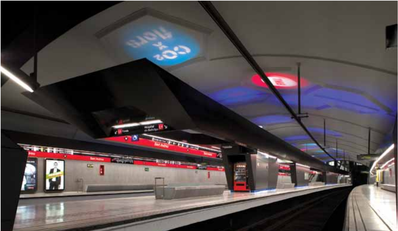
The metal structure, almost 80 meters in length, supported by just three points, allows more interior space under the vault, such as signs, vending machines or the projectors that illuminate the vault.
