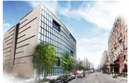
Huaku-Dazhi Building TAIPEI, TAIWAN PGS. 34-35
